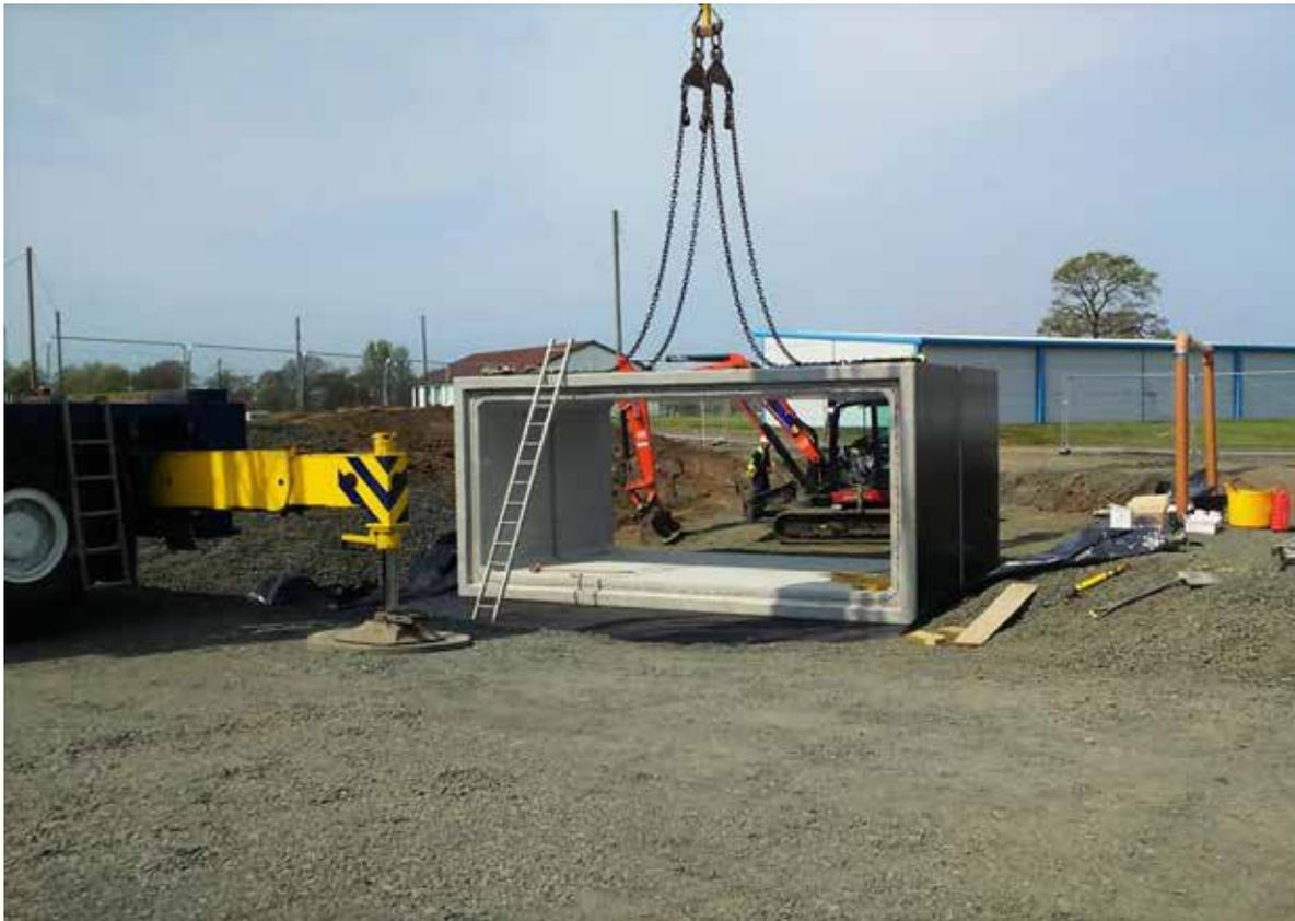
The first culvert is lowered into place
