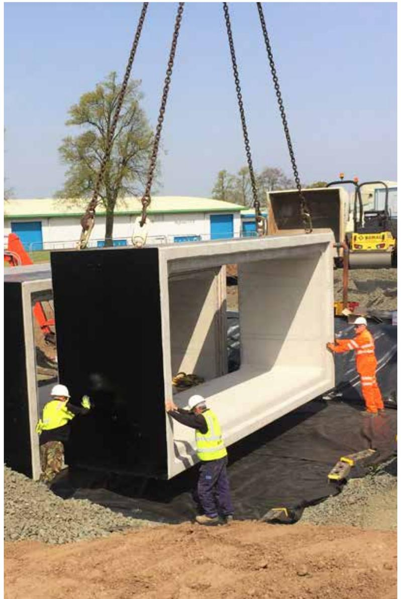
Contractors guide the second culvert into place (top). The finished underpass and livestock bridge (right)
